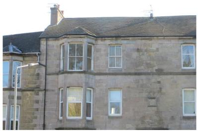
Figure 24 Levengrove Terrace, original windows with replacements and concrete tile roof replacement; central chimney also looks to have been removed
