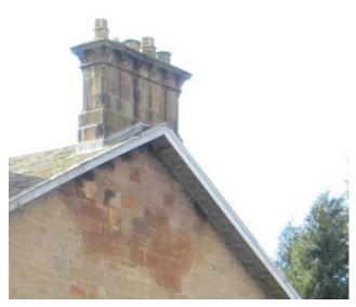
Figure 23 Water penetration below chimneys is seen on a number of properties
