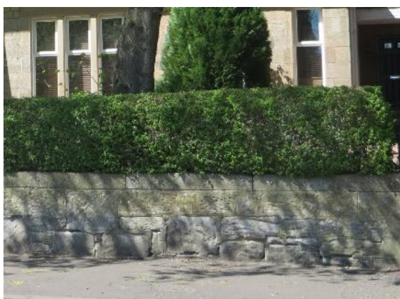
Figure 14 Left: Boundary wall with erosion. Right: Boundary wall with salt efflorescence.
