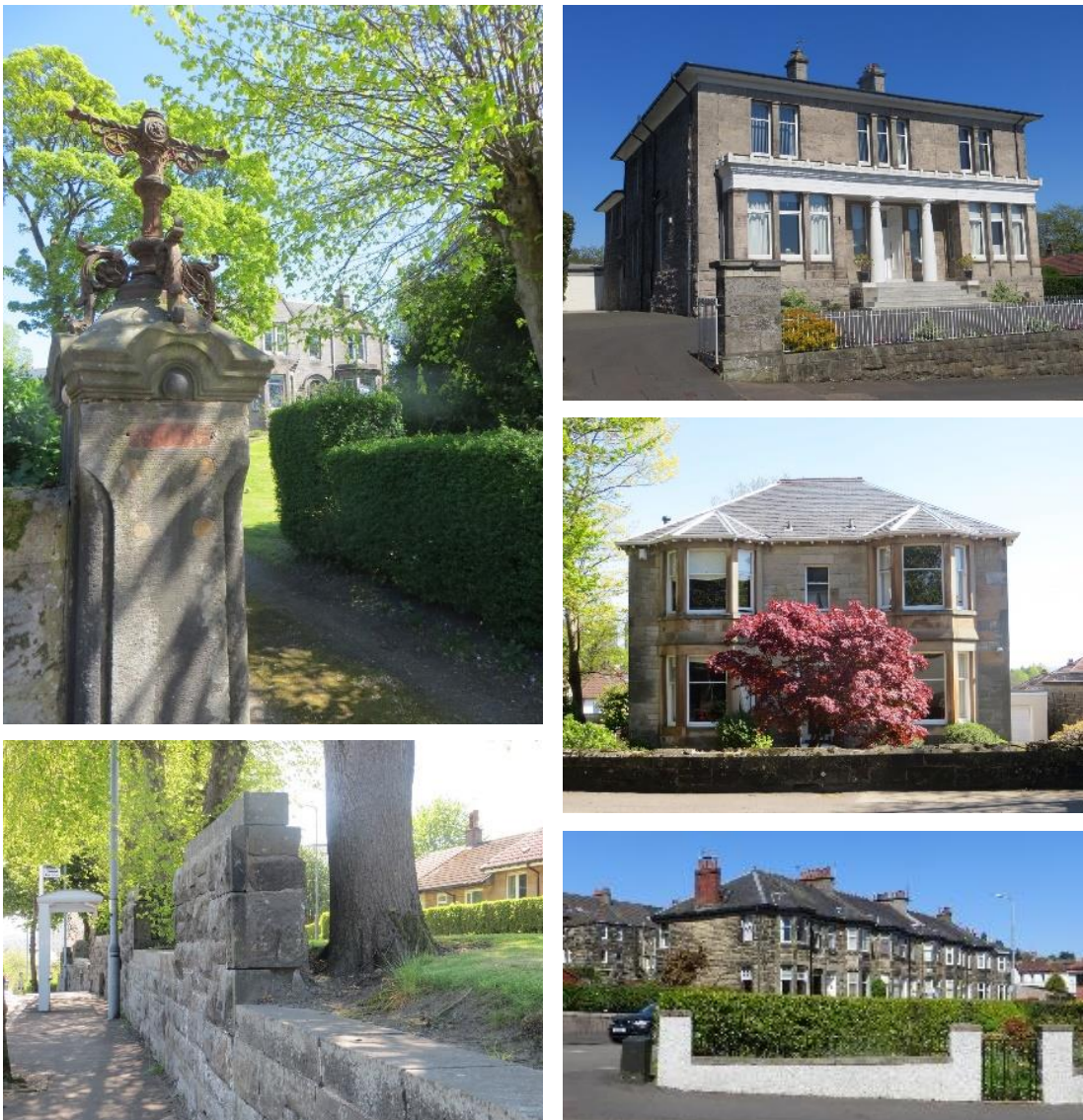
Figure 17 Clockwise from top left: 36 Park Road with carved stone entrance piers and remains of cast iron lamp standards; Melbourne House, the single Victorian survivor on Regent Street; 48 Duntocher Road, sits opposite Overtoun Road at the entrance to the conservation area; Edwardian terraced houses on Methven Street with Maxwell Street beyond; surviving boundary wall to the former villa of Uladh Tower.
