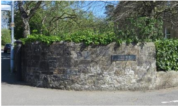
Figure 17 Lusset Road – curving stone wall to Craigview with conservation area signage and original iron gate post
