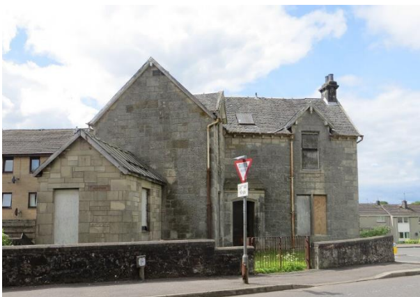
Figure 19 No. 2 Station Road.
