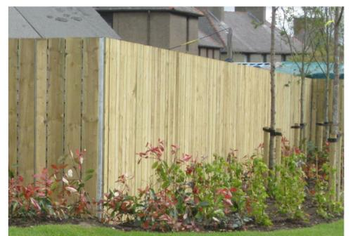
1800mm Timber screen fence with galvanised posts and frame.
