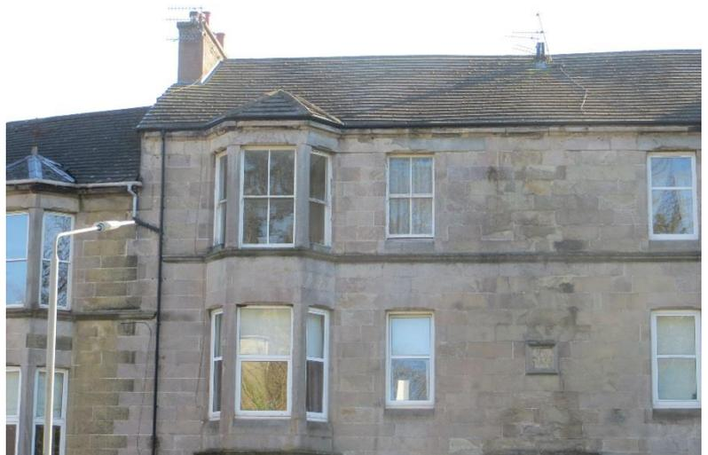
Figure 24 Leven Grove Terrace, original windows with replacements and concrete tile roof replacement; central chimney also looks to have been removed
