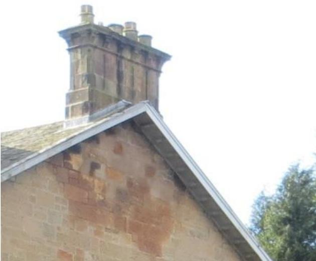
Figure 23 Water penetration below chimneys is seen on a number of properties
