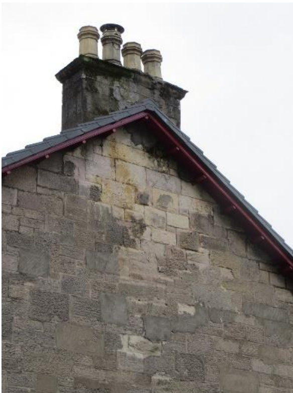
Figure 21 Stone erosion at gable chimney and defects to chimney above.
