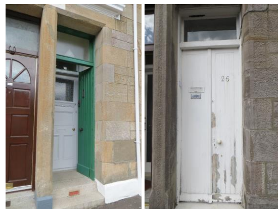
Figure 13 Original door design on Buchanan Street.
