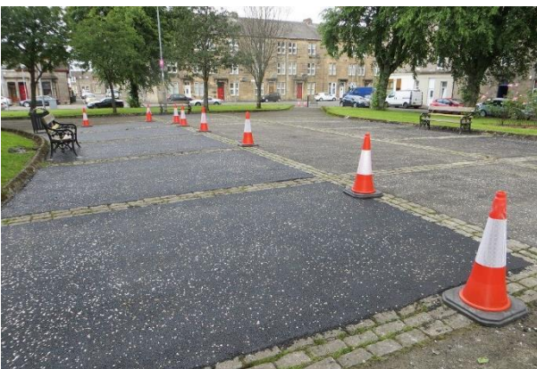
Figure 16 Knoxland Square: resurfacing underway in June 2017.
