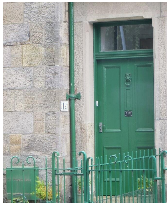
Figure 14 Door on Knoxland Terrace.
