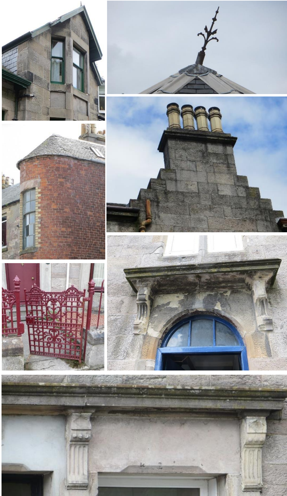
Figure 15 Clockwise from top left: Bay window with original timber sash and case windows, south side of Knoxland Square; finial detail; stepped front chimney on Knoxland Square tenement; corbelled lintel over tenement entrance, Knoxland Square; lintel detail on Victoria Street; decorative cast iron gate on Victoria Street terrace; red brick stair tower to the rear of Knoxland Square with original curved timber sash and case windows and Scots slate roof.
