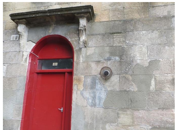
Figure 24 Poorly executed cementitious stone repairs, stone erosion to door lintel, and obtrusive vent.
