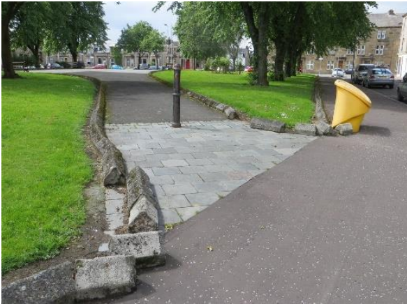
Figure 18 Knoxland Square – mixture of tarmac and paving surfaces, concrete kerbs in poor condition and loose.
