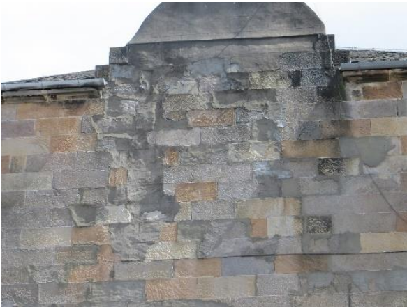
Figure 20 Stone erosion at gable chimney poorly repaired in cement.
