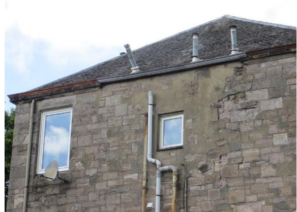
Figure 23 example of window replacement in non-consistent design and opening method and gable chimney removal with poor repair below.
