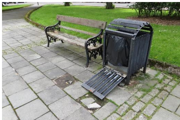
Figure 17 Knoxland Square: paving, bench and waste bin in poor condition.
