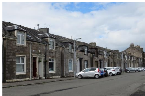
Figure 25 Above: Tenement block on Castlegreen Street – very similar to the Knoxland Square block. Below: Semi-detached houses on Wallace Street to the same design as Bruce Street.
