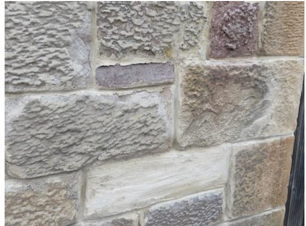
Figure 22 Stone erosion at gable poorly repointed in cementitious mortar and plastic stone repair.
