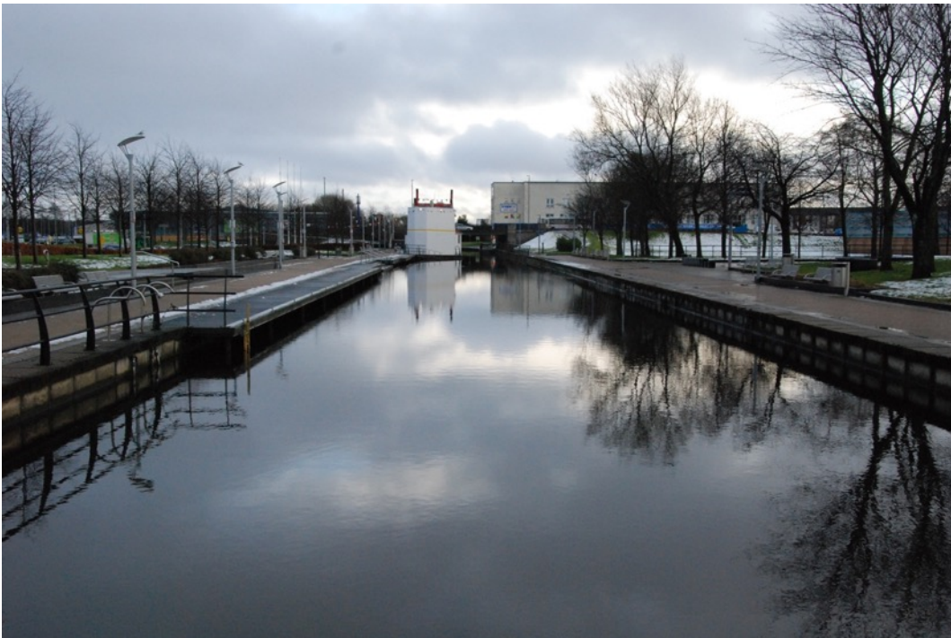
Forth and Clyde Canal in Clydebank Town Centre
