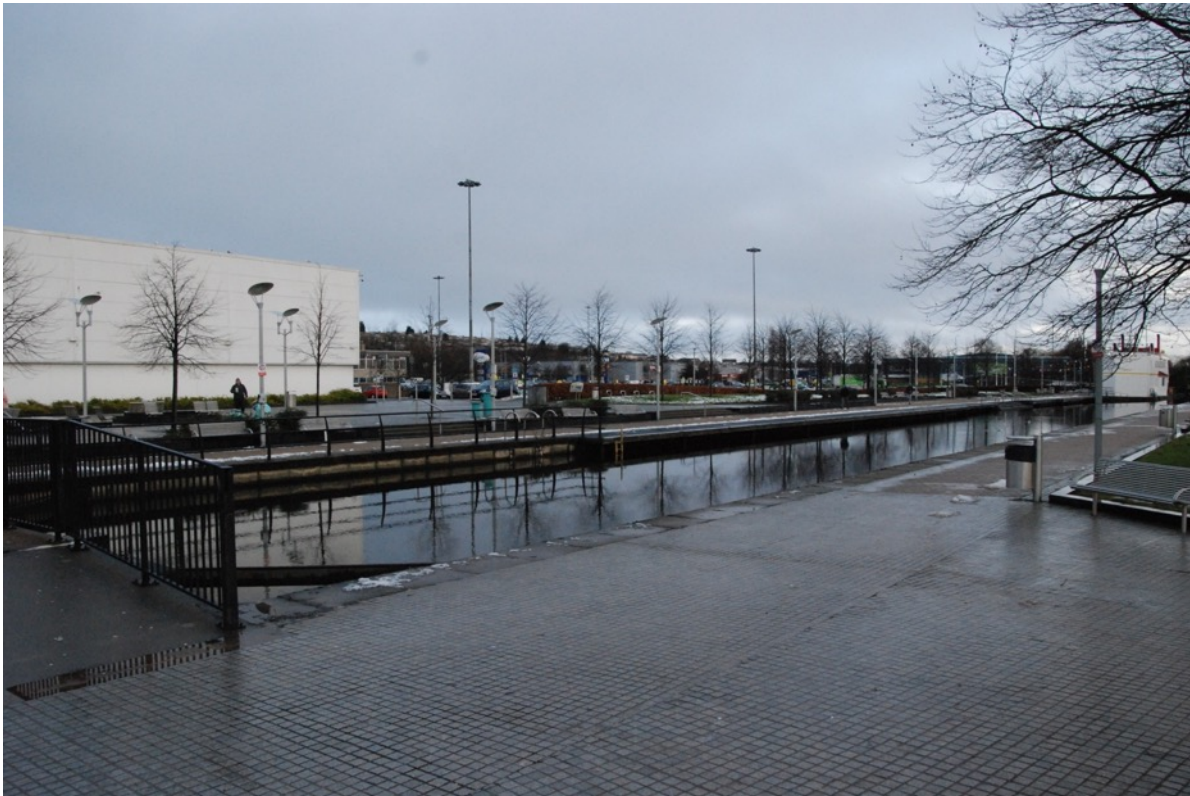
Looking towards the North bank of the canal
