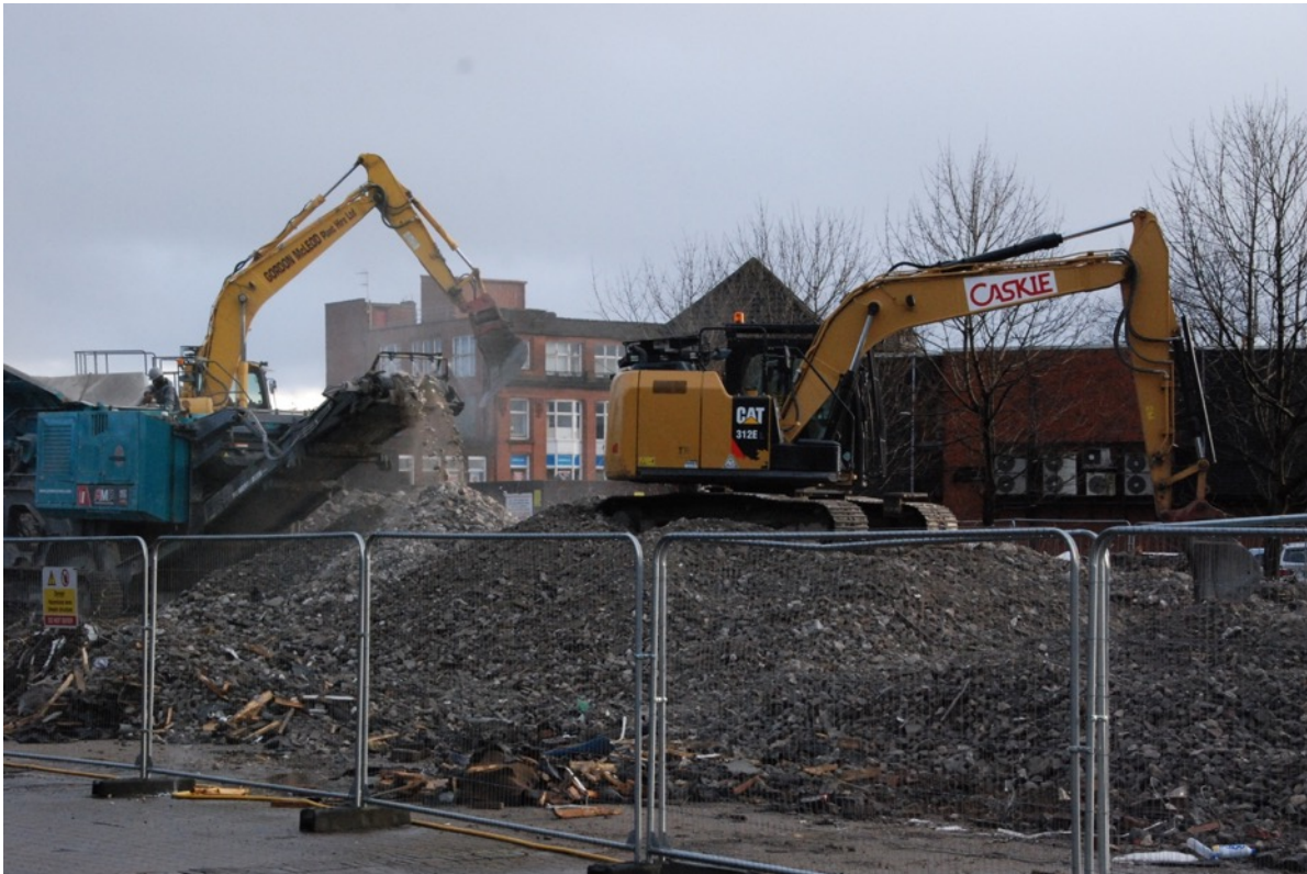
Site clearance on Rosebery Place
