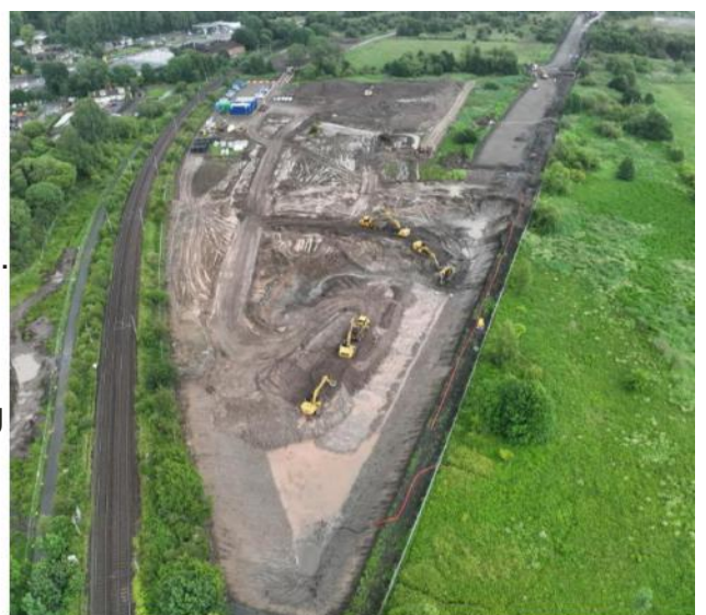
Earthworks preparation of the Casting Yard
