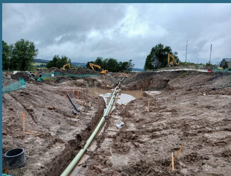
Visual of the gas main diversion, showing new pipeline being laid and welded.
