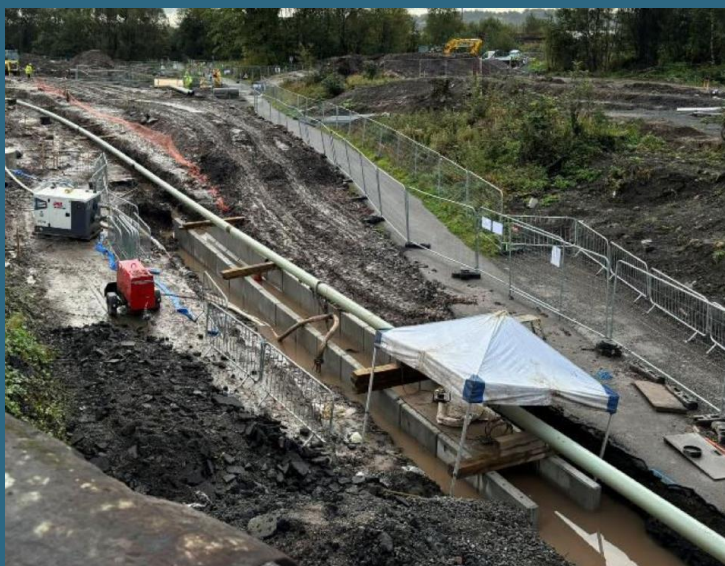
Visual of the installation of the reinforced concrete protection units for gas main diversion.
