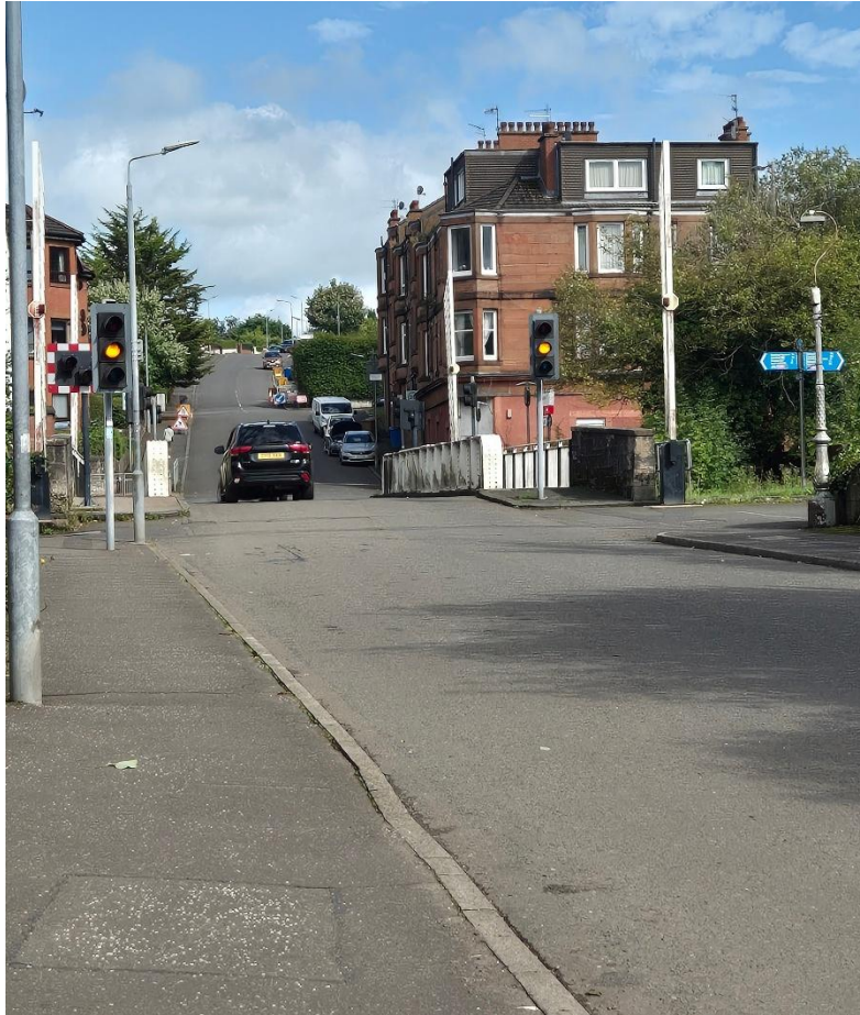
Pavement towards canal path – no dropped kerb
