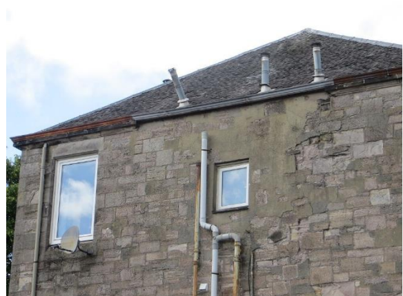
Figure 23 example of window replacement in non-consistent design and opening method and gable chimney removal with poor repair below.
